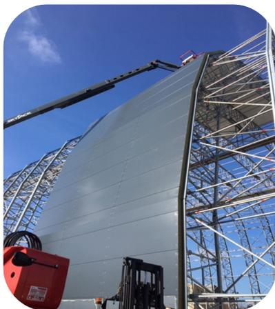
This provided a sound structural member with which to affix the horizontal cladding panels (again shown clearly in the images adjacent).
